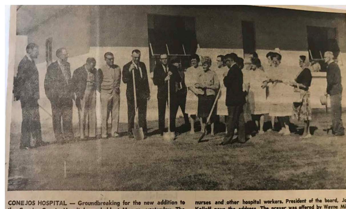
CONJOS HOSPITAL — Groundbreaking for the new addition to the Conejos County Hospital was held at 11 a.m. yesterday. The new addition, made possible by the $100,000 bond issue approved last spring will provide 15 additional beds, a new obstetric department, additional office space and a lobby. Present for the ceremony were members of the hospital board, staff doctors, nurses and other hospital workers. President of the board, Joe Kelliff gave the address. The prayer was offered by Wayne Miller, hospital administrator. Men shown above, left to right are Dr. Dale Thomas, Otha Baggett, A. Mandel, Ben Kuchel, Alamosa, contractor for the addition, Kelliff, Dr. V. Johnson and Miller. Completion is expected to be May 15. (Watersburg Photo)
